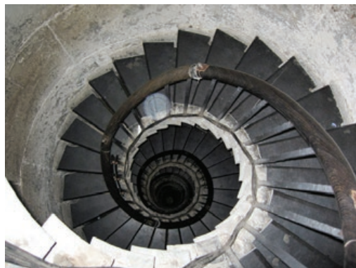
A typical staircase in the Tower of London.
